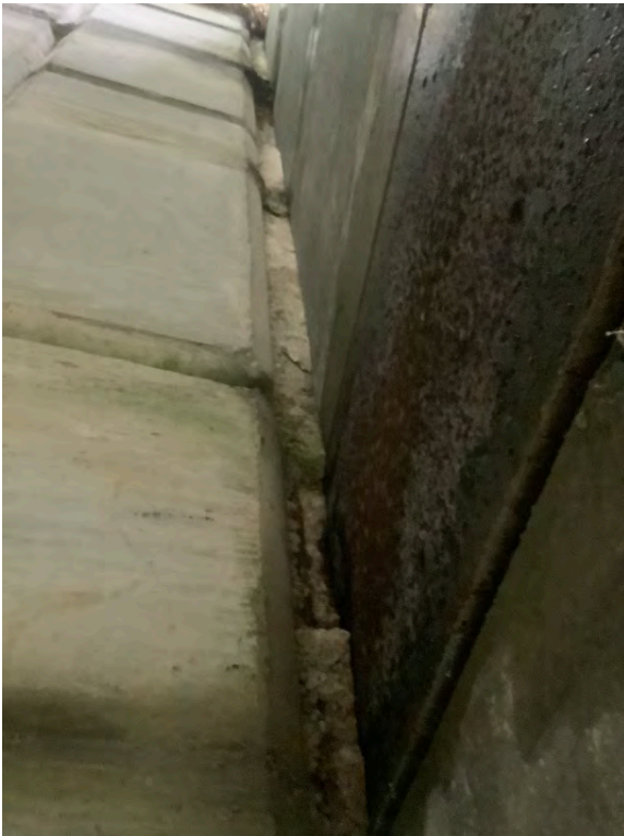
Right Bank Abutment when facing downstream
